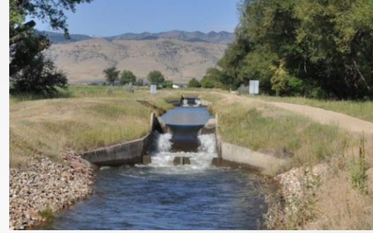
Figure 6 Canal drop structure
