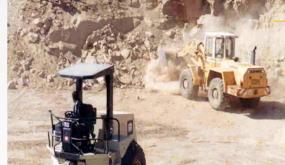
Figure 5 Halhal dam construction, 1997
